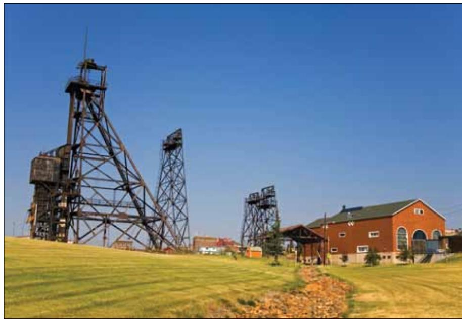
**Figure 5.** Underground mine head frame and hoist room.
