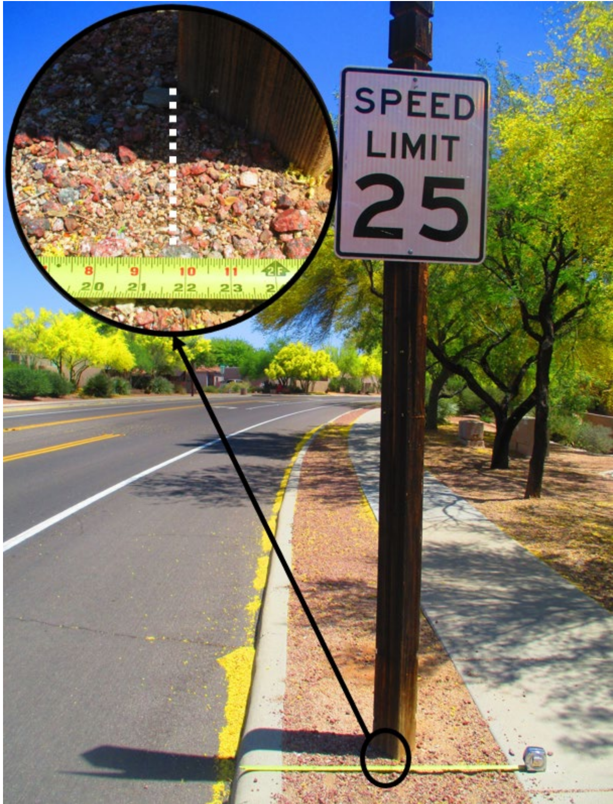
Figure 10. Measuring CDIST, this sign support has a curb offset of 1.8 feet (22 inches).
