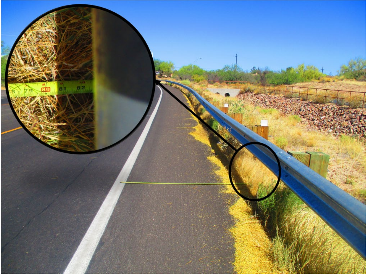
Figure 5. Offset measurement of longitudinal barrier, this offset is 6.9 feet (83 inches).
